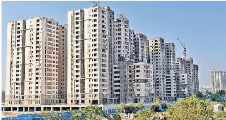
MAKING IT MANDATORY: The rules, which came into effect from August 4, specify that the builders should register the project and its specifications with Rera. — Photo: Hrudayanand
